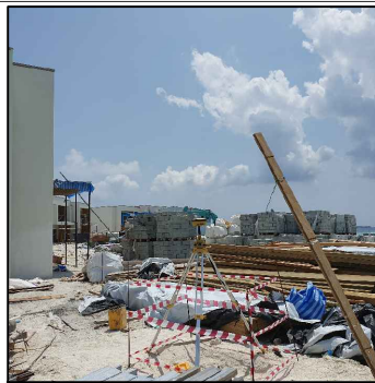
NORTH VIEW Distance 5m, height 1.5m
